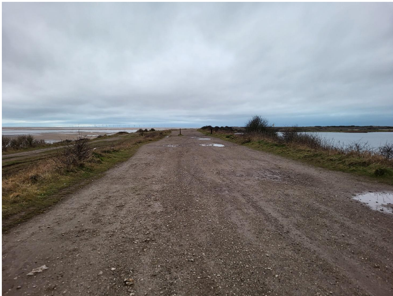
Figure 8.3 The excessively wide road along the sea wall (Photo taken in February 2023 looking south east)
