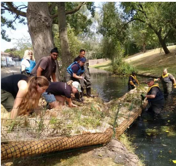
Figure 10.8 Thamesmead volunteer programme building floating reedbeds
