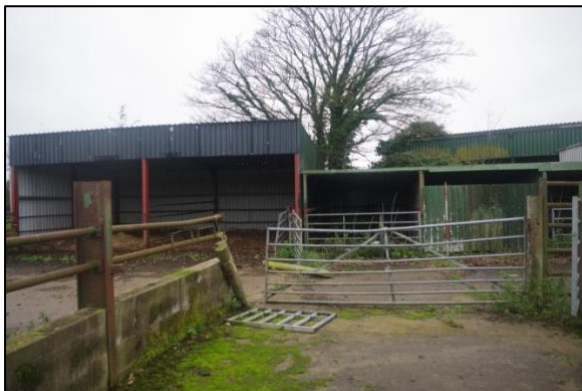
Figure 10. Redundant agricultural buildings
