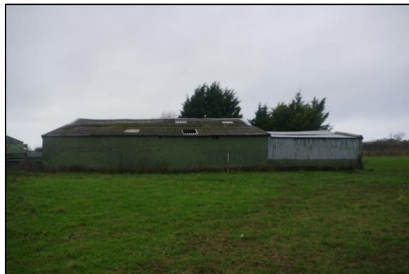
Figure 11. Barn in Field 1
