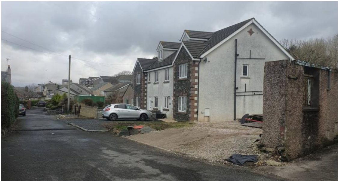
(Fig.11 – View looking North on Cleator Street)
