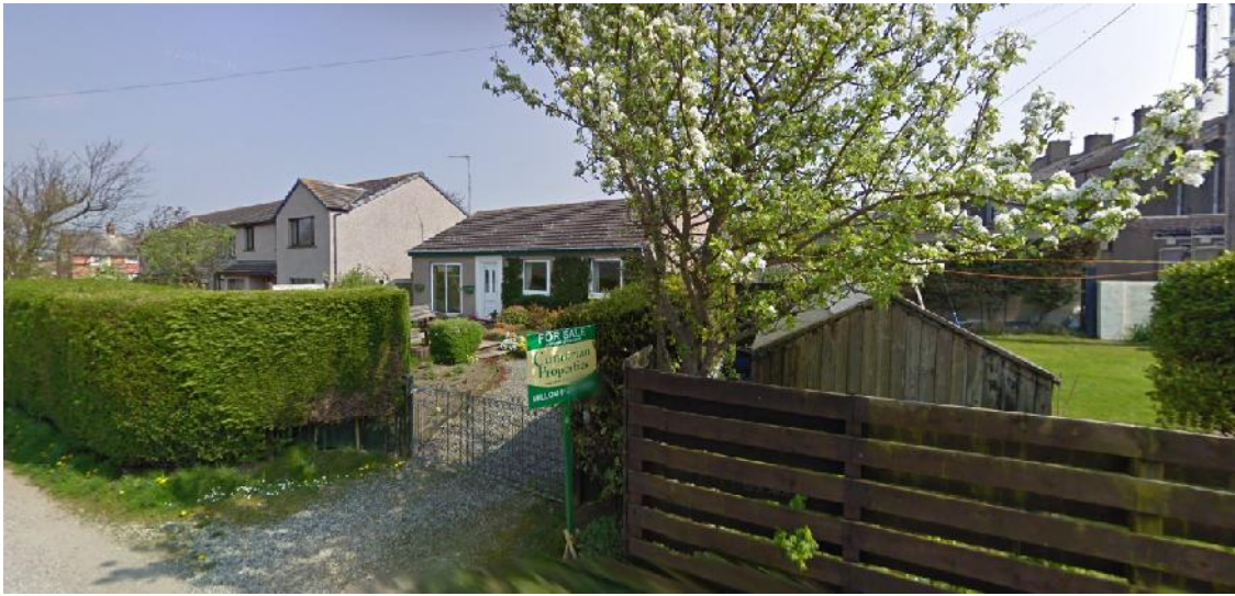
(Fig.10 – Single storey bungalow & 2 storey dwelling to the West of the Application site accessed from Church Walk)
