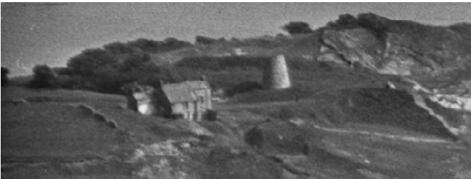
Aerial image (circa 1930) depicting the former 'offices' (left) and windmill (right).
