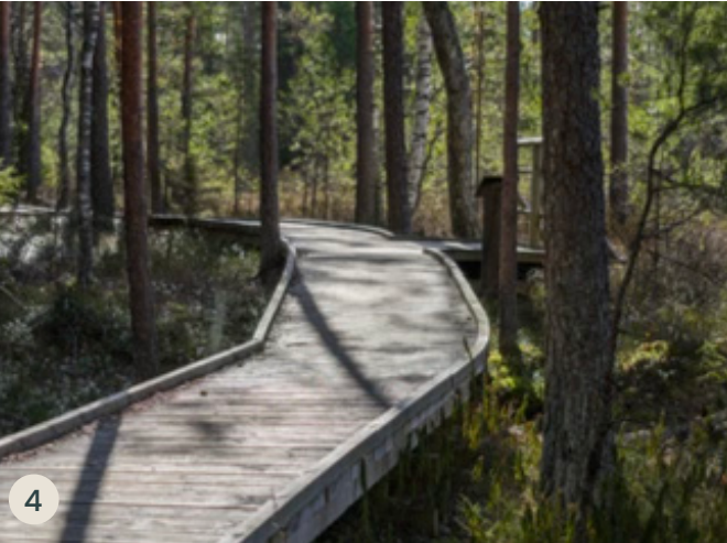
Raised Timber Boardwalk
