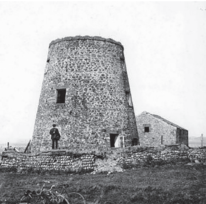
The Old Windmill, Walney Island with only masonry structure remaining (date unknown).
