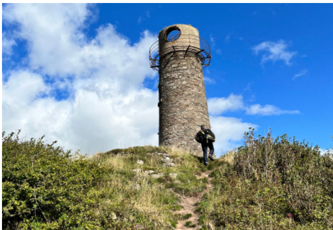
Poor access to heritage assets
