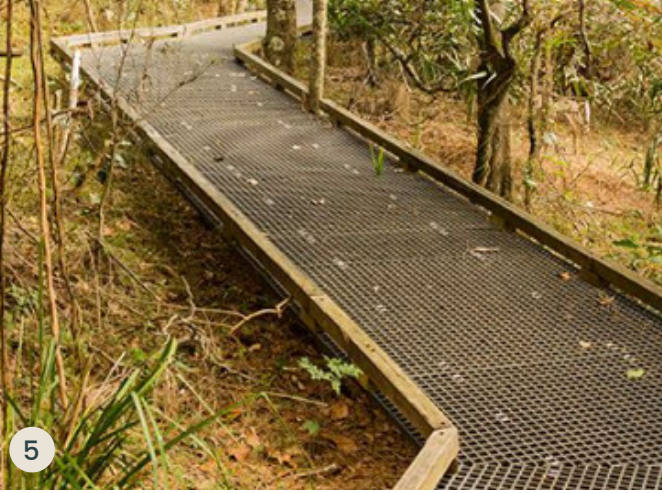
Raised Steel Walkway
