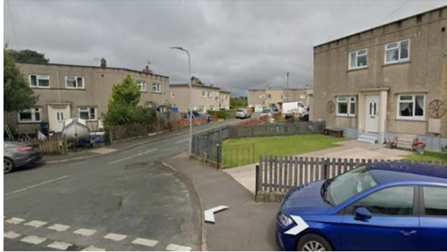
1 Existing houses - Dent Rd to south of site
