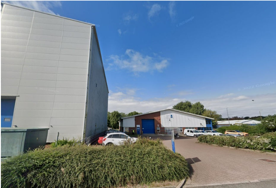
View from East, toward location of extension
