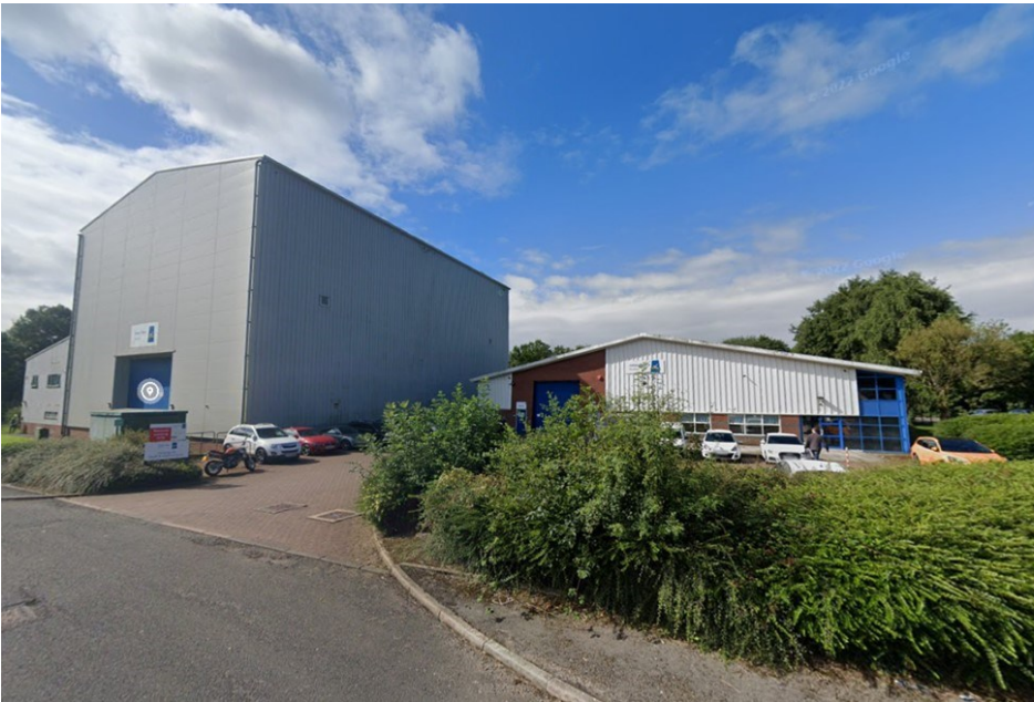
View from North East, toward location of extension
