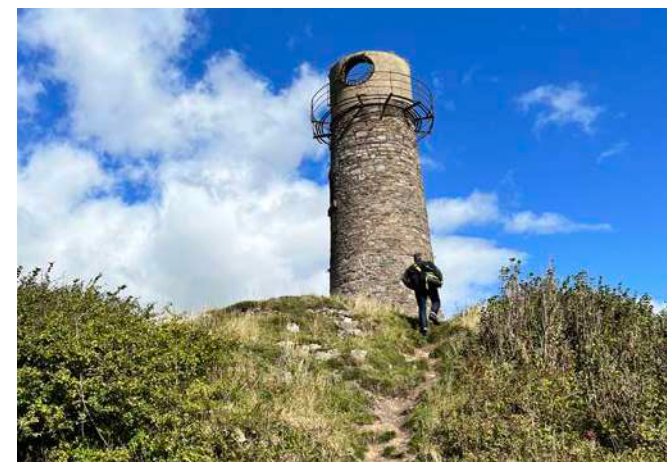
Poor access to heritage assets
