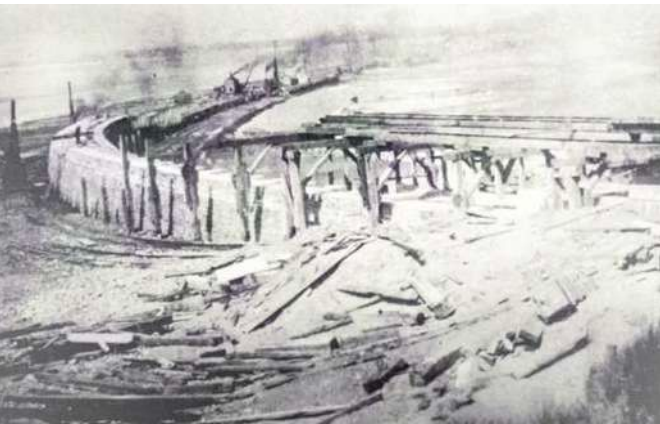
Inner sea wall construction
