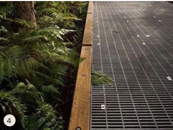
Steel Walkway with Timber Edging
