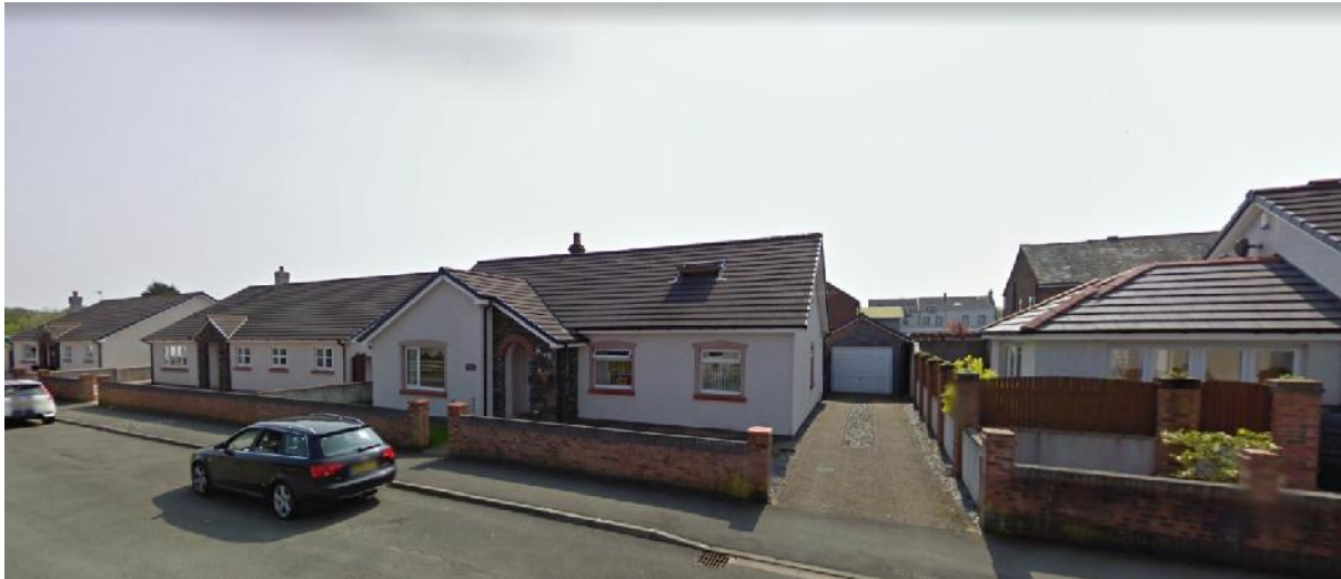
Fig. 20 – Single Storey detached dwellings along Millom Road)
