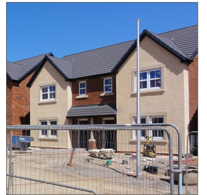
Rendered gables and congruent window surrounds. This key 'Spencer' housetype (under construction within Phase II) will also be used within Phase IV
