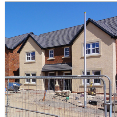
Rendered gables and congruent window surrounds. This key 'Spencer' housetype (under construction within Phase II) will also be used within Phase IV
