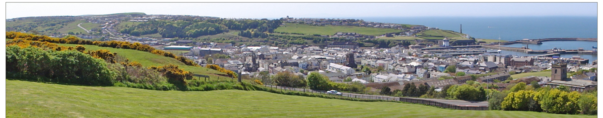
Cross-town view highlighting render finishes and slate roofs, creating a generally united and coherent townscape
