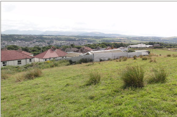
Fenced area 'land grabbed' by an adjacent occupier along Valley View Road. Proposed planting will help screen this area
