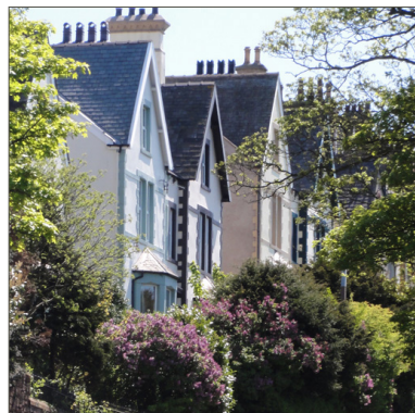
Victorian dwellings often incorporate steep, decorated eaves and gable elements
