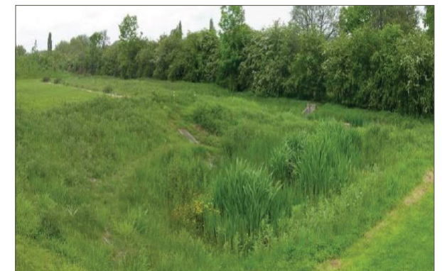
Design cue - south eastern SUDS infiltration area / dry basin
