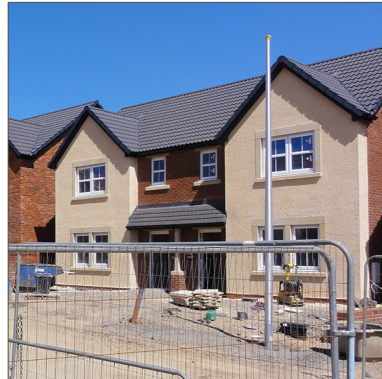
Rendered gables and full surrounds. Story's 'Spencer' house type
