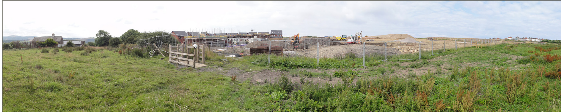
Panoramic view looking west across entire westerly boundary to Phase IV with High House to the south and temporary kissing gate access to the PROW running between Phases II and III of the developing Edgehill Park to left of centre. Rendered dwellings to the southern edge of Woodhouse visible to the north (right)
