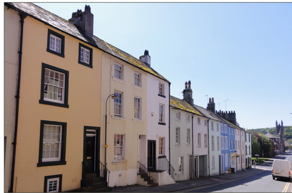
Most buildings in the town centre present a consistent street façade and located to the front of building plots in line with Lowther's 1699 regulations. Undulating eaves result largely from underlying topography
