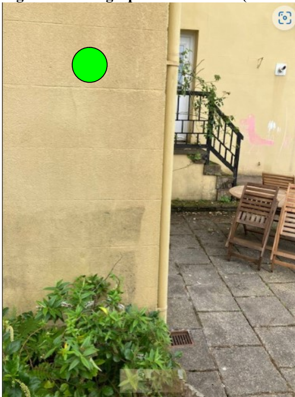
Figure 4: Photograph of Gable End (Photo 1)
