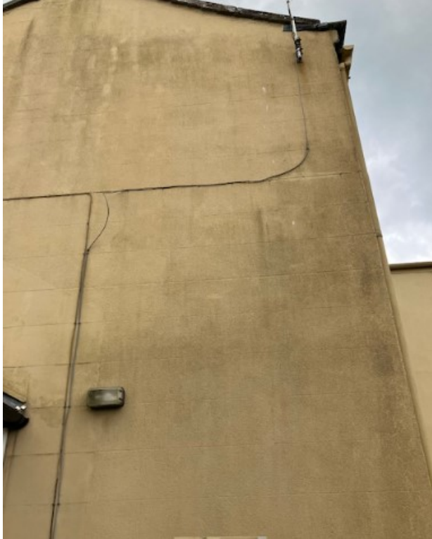
Figure 5: Photograph of Gable End (Photo 2)
