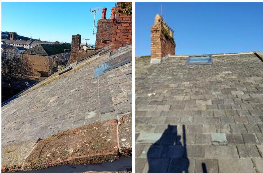
Site photos 8 and 9 of new replacement roof with dormer removed.
