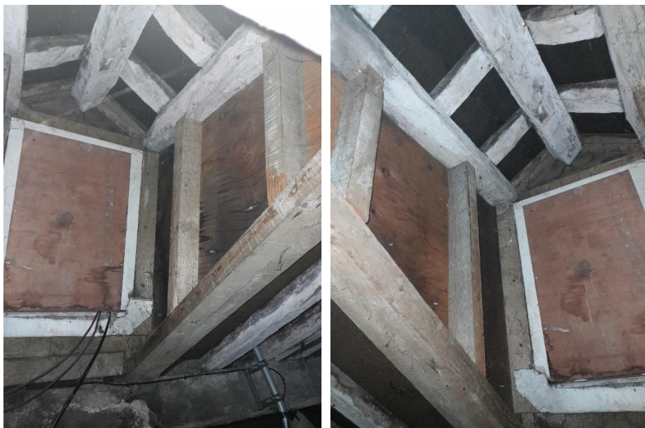
Site photos 8 and 9 of new replacement roof with dormer removed.
