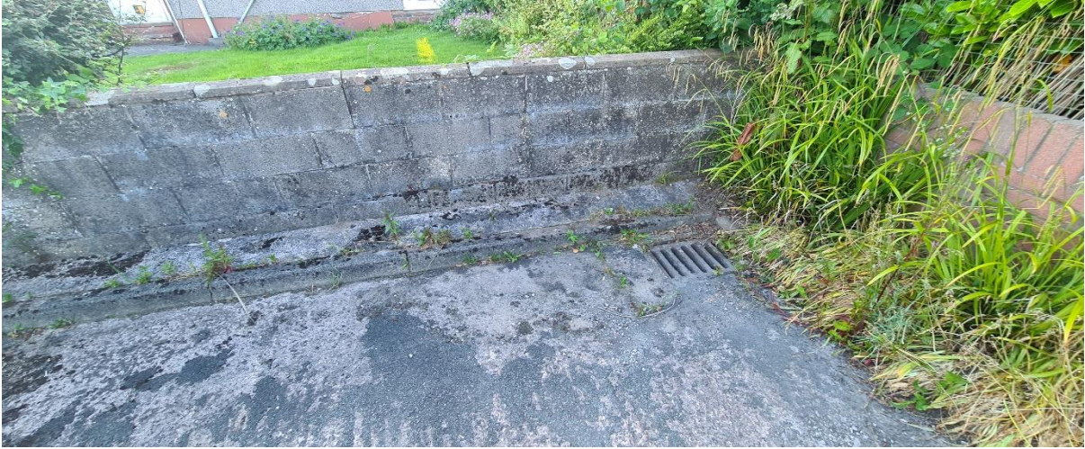
Image B – Surface water drain.
