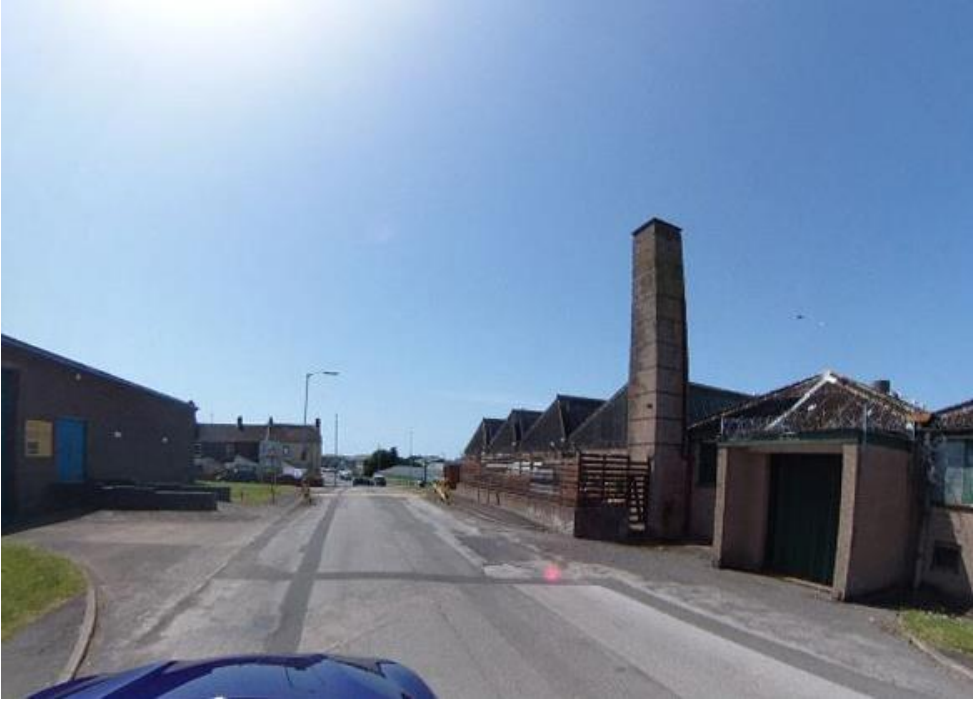
5 - Leconfield Industrial Estate –Existing main access road to be retained and improved
