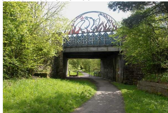
C2C Phoenix Bridge
