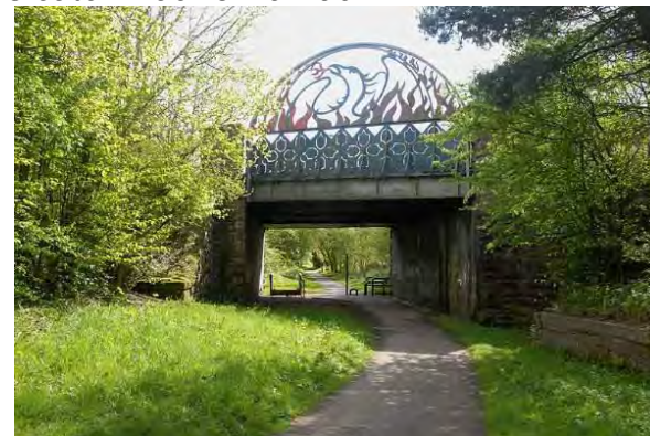
C2C Phoenix Bridge
