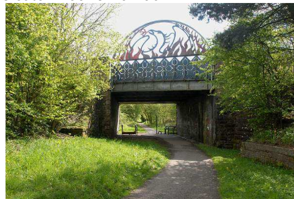
C2C Phoenix Bridge
