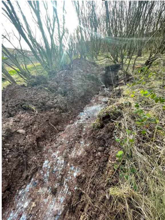
Figure 13: Area of slit trenching around Shaft 008.
