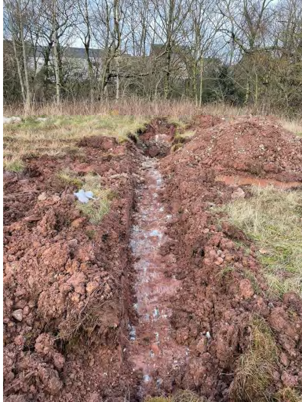
Figure 11: Area of slit trenching around Shaft 006.
