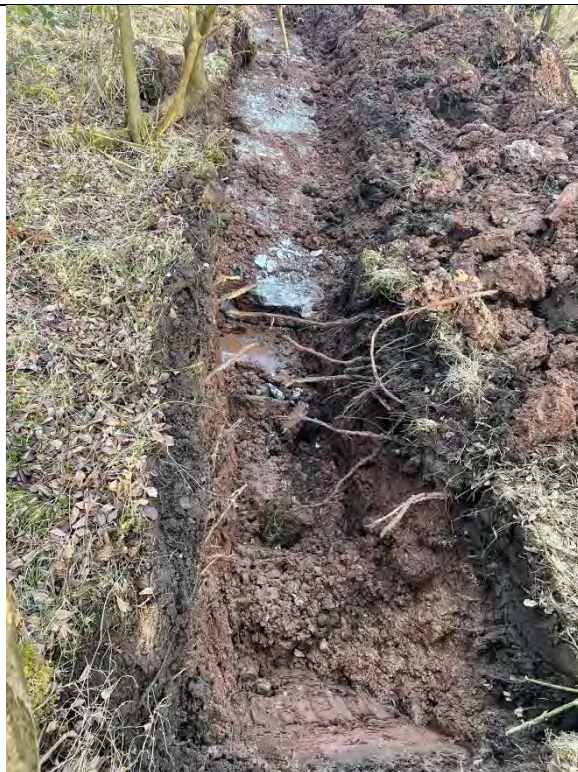
Figure 12: Area of slit trenching around Shaft 008.
