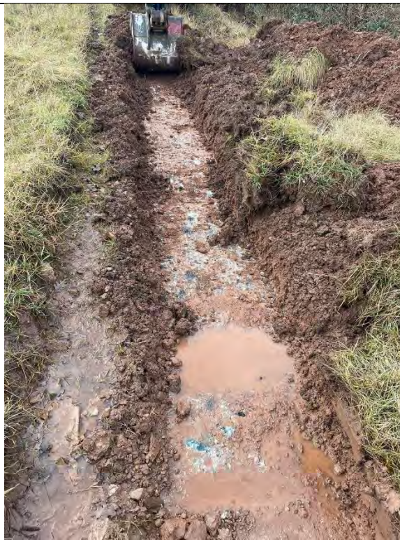
Figure 10: Area of slit trenching around Shaft 006.
