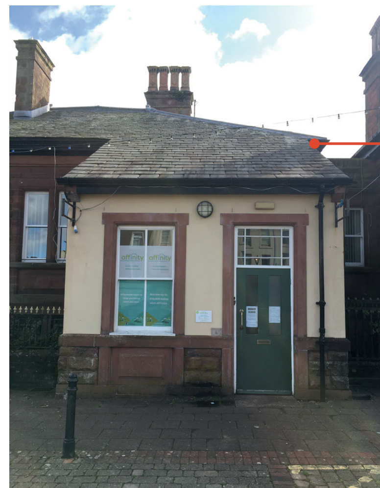
Fig 33 Accessible entrance on Jacktrees Road Elevation. No visual distinction between original building and recent additions.
