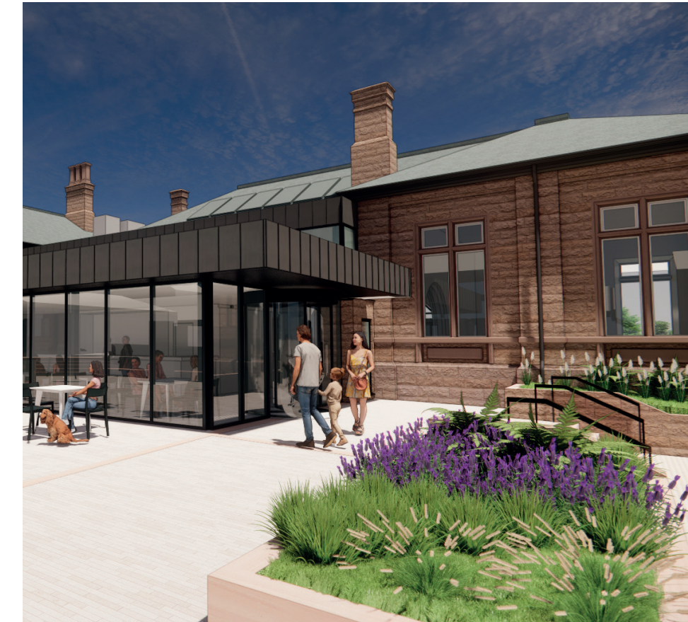
Fig 30 External view of extension showing level changes for accessible route.
