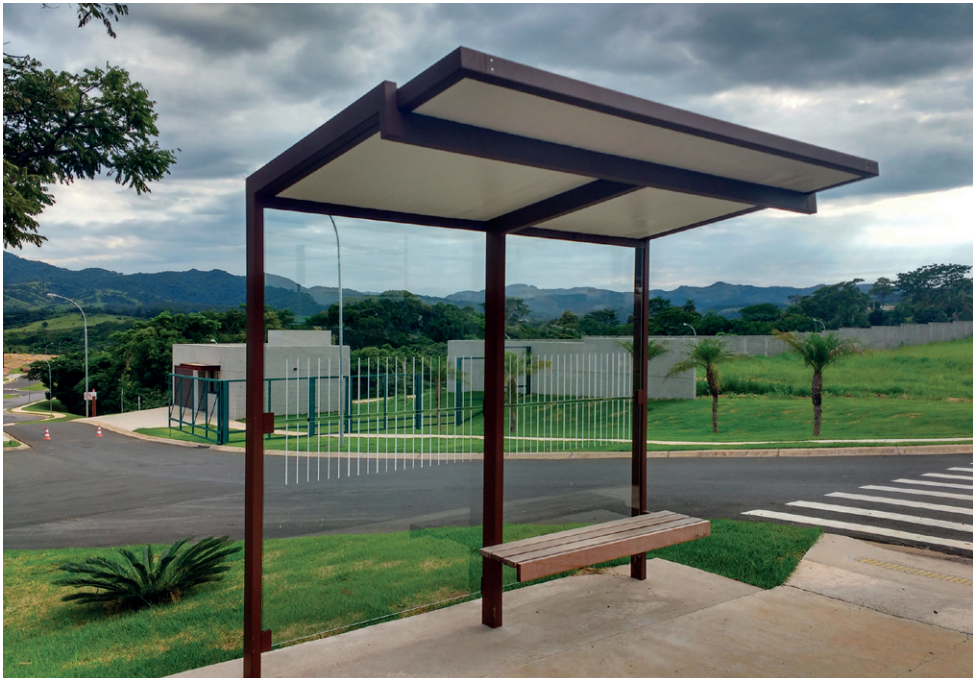
Bus shelter with green roof
