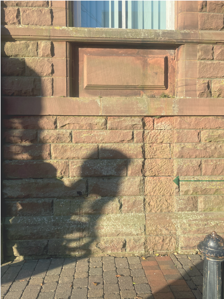
FIG 08 Site image showing the Town Hall building, viewed from the gap between this and the library.
