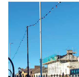
Existing columnar and festoon lighting
