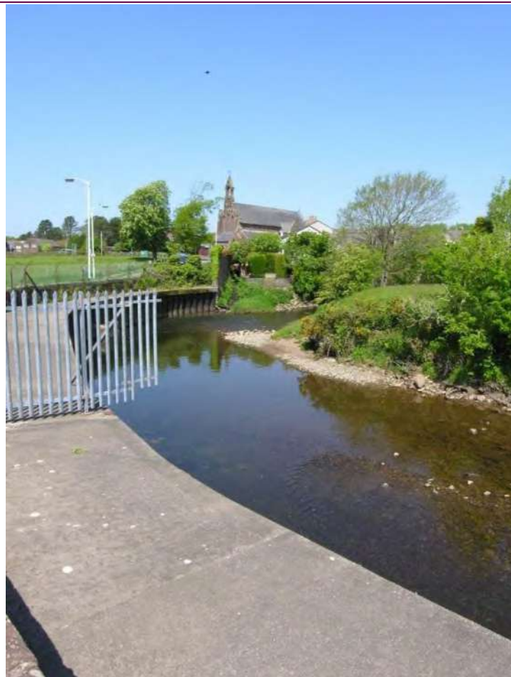
Photo 1 – Hard flood defences between 1896 & 1726
