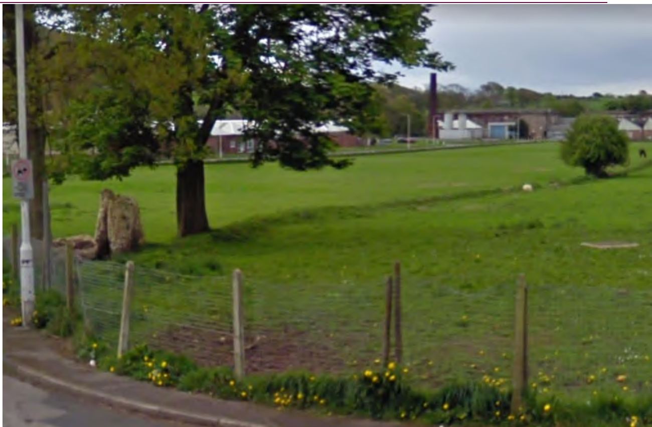
Photo 2 – Raised mound and kerbs along overland flood route
