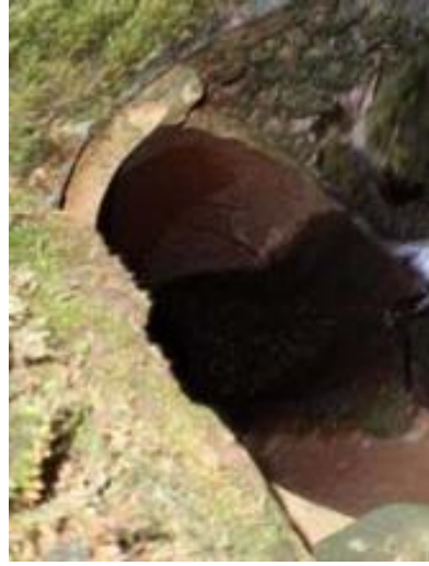
U/S broken 18" clay pipe
