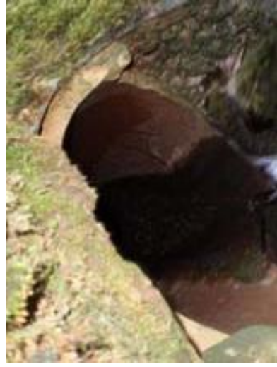
U/S broken 18" clay pipe
