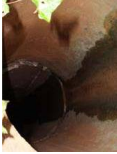
D/S 18" clay pipe flowing clear #1
