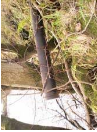
U/S broken 18" clay pipe
