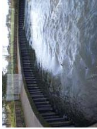
Sheet pile FI showing minor distortion But flood wall well protected by concrete berm
