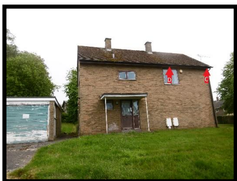
Plate 4: Roost C & D (Building 9).
