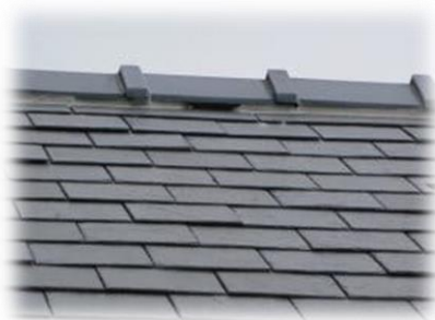
Plate 10: Example of bat ridge access
