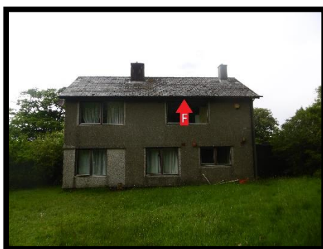
Plate 3: Roost F (Building 5).
