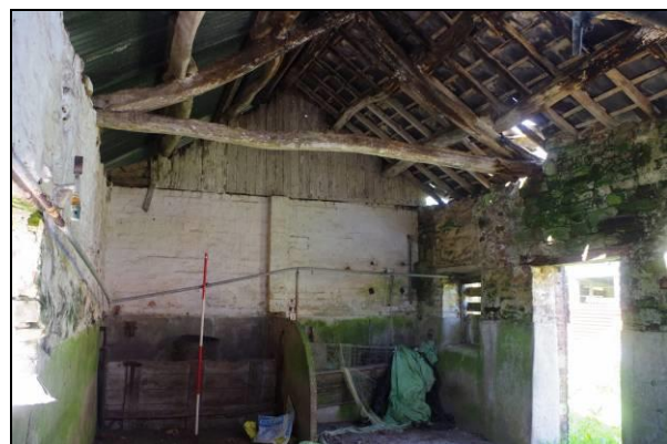
Figure 13. Interior to Room 2 looking north
