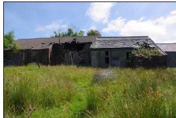
Figure 37. Western elevation Buildings 3 to 5
