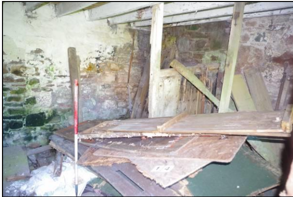
Figure 34. Room 14, a stable, Building 6
