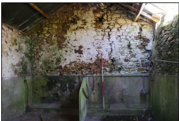
Figure 16. Northern end of Room 3, Building 2
