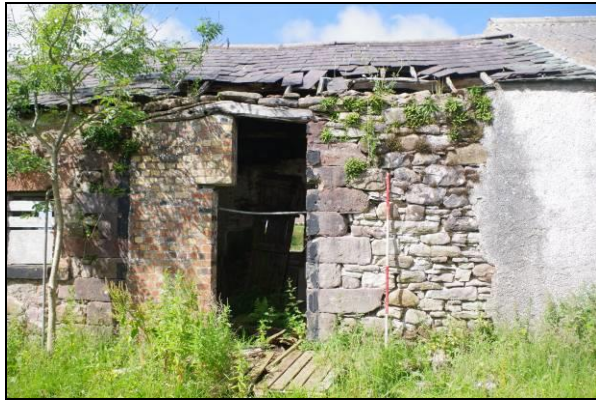
Figure 15. Entry to the threshing barn, Building 2
