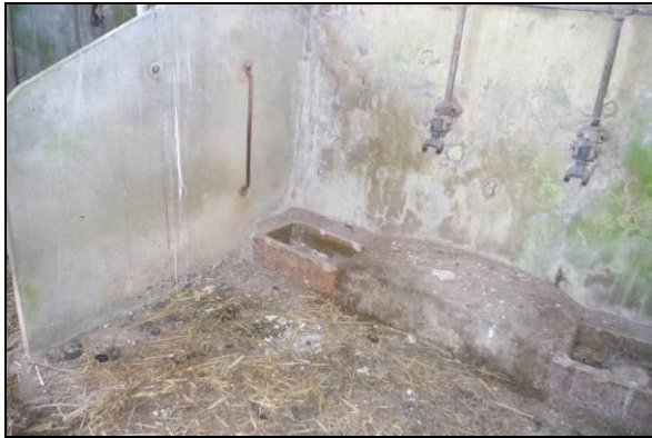
Figure 10. Trough in Room 1
