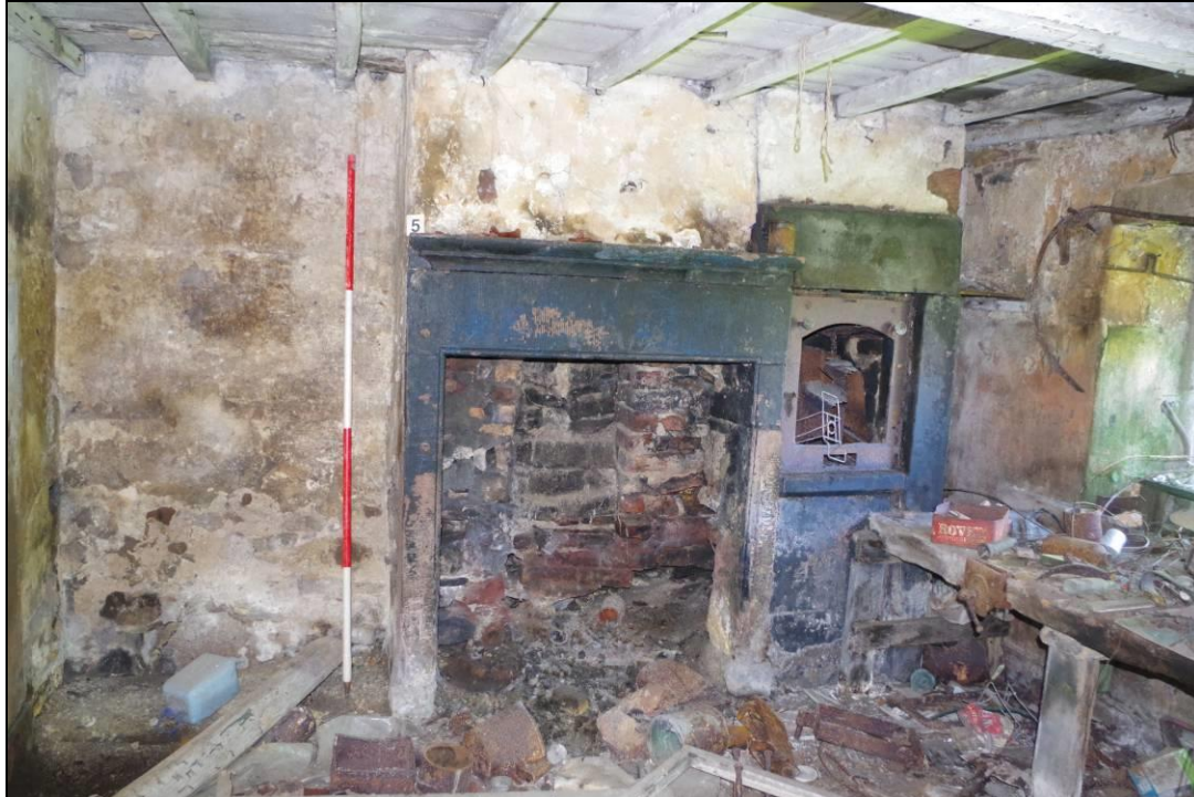
Figure 22. Room 5, the kitchen, Building 3
