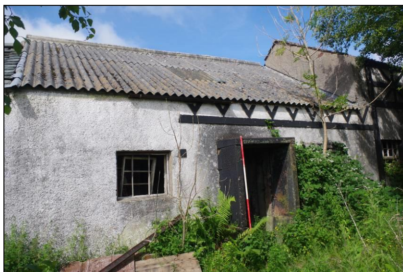
Figure 19. Facade of Building 3
