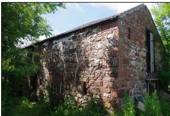
Figure 32. Elevation of Building 6
