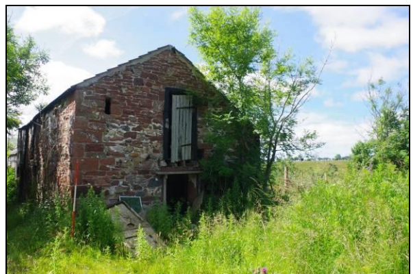
Figure 33. Northern gable end of Building 6
