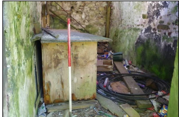
Figure 31. Room 12, a store, Building 5
