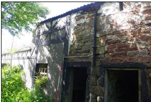
Figure 27. Elevation of Building 4
