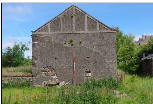
Figure 6. Southern gable end of Building 1
