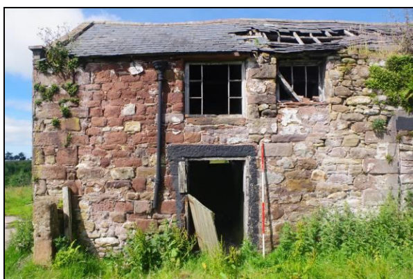
Figure 5. Eastern elevation of Building 1
