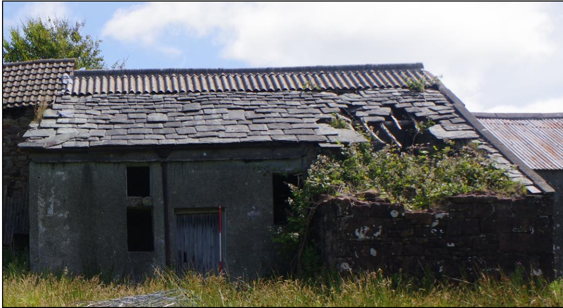
Figure 23. Outshut to Building 3
