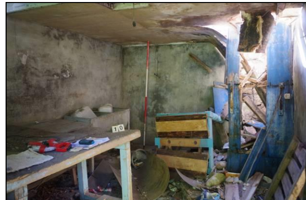
Figure 28. Room 10, a store, Building 4
