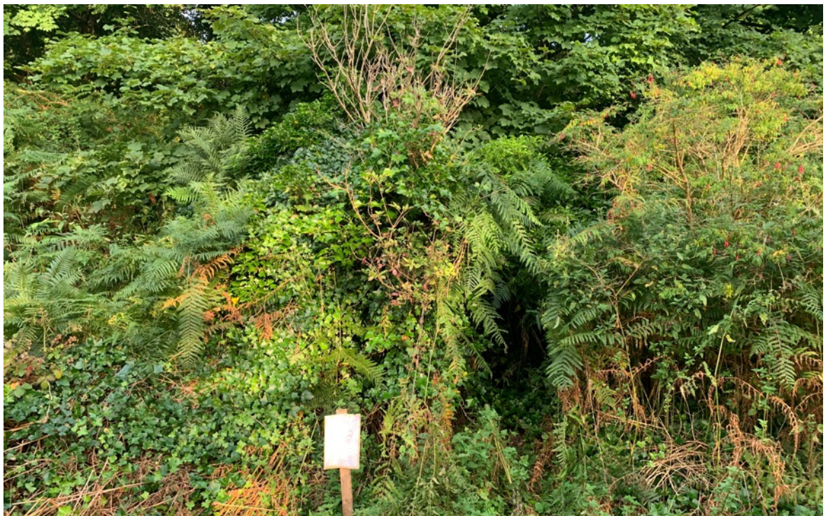
Photograph 1. Exterior of outbuilding
