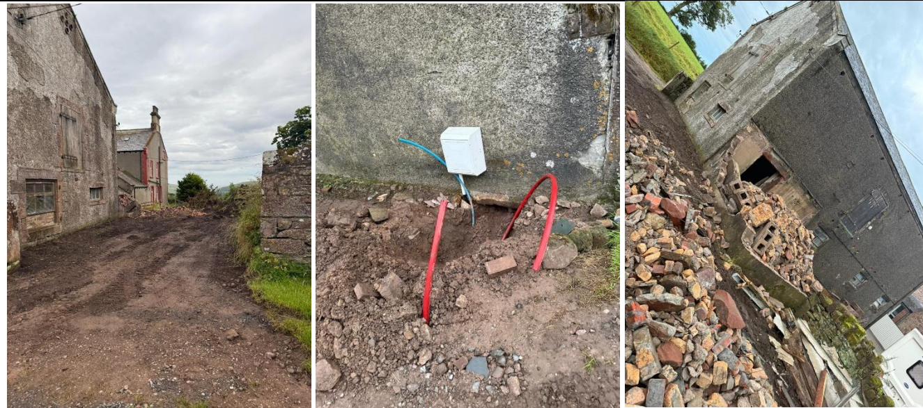
Figures 1-3 above showing evidence of demolition and ground works on site.
