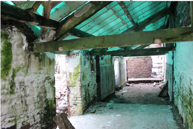
North wing looking west with new roof on existing truss
