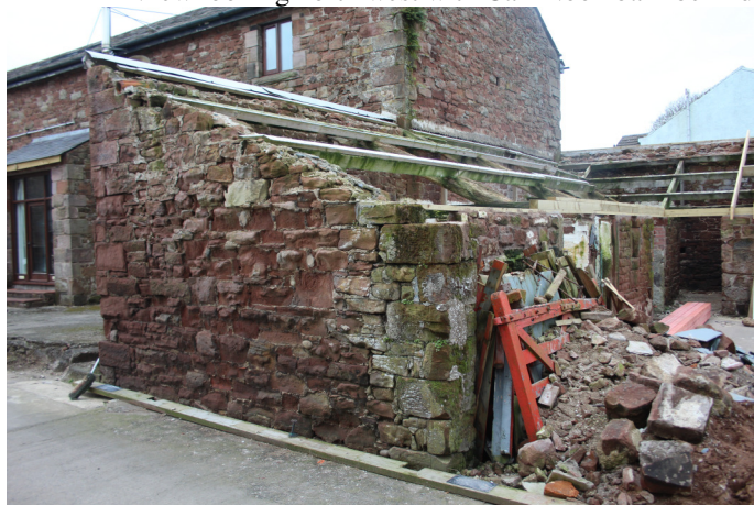
View looking north west with Calf Nook barn behind
