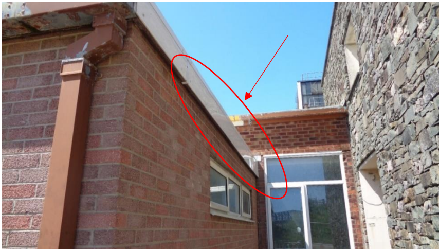
Photograph 3-1: Exit location on the northern face of Building F4b
