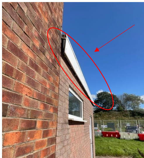
Photograph 3-2: Exit location on the southern face of Building F4b
