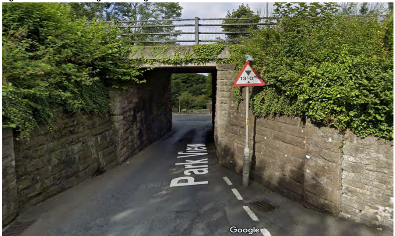
Figure 21 Park View Bridge/Narrowing
