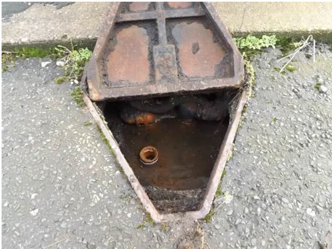
PLATE 4 – MANHOLE COVER WITH ACCESS TO UST AT REAR OF FUEL PUMPS
