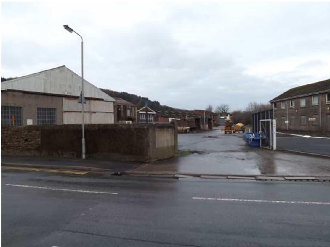
PLATE 2 – VIEW OF THE SITE LOOKING NORTH FROM COACH ROAD
