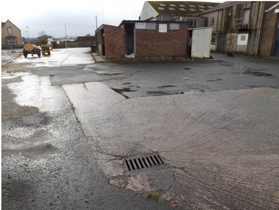
PLATE 3 – EXISTING BUILDING CONTAINING FUEL PUMPS
