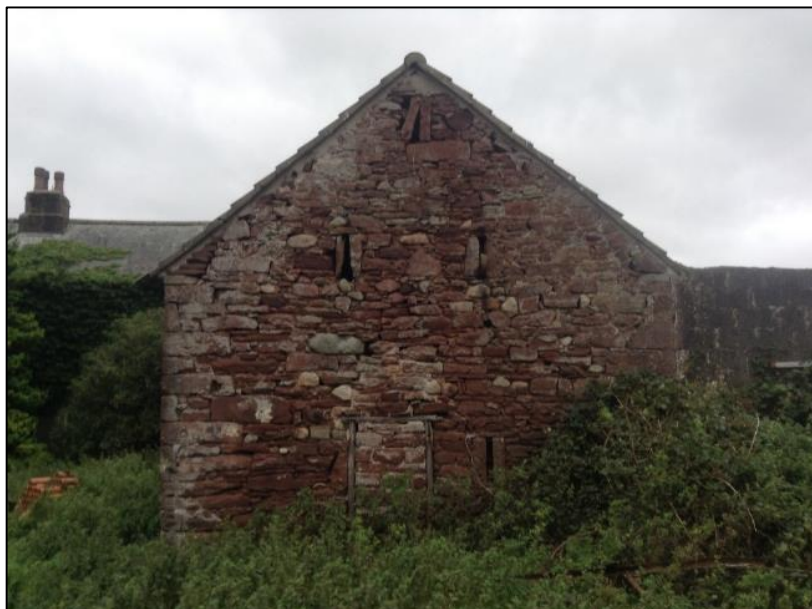
Photo 8: Eastern elevation of Building 2. Numerous gaps in the stonework across the whole elevation.
