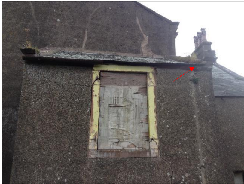
Photo 3: Western elevation of Building 1. Gaps in exposed stonework at soffit
