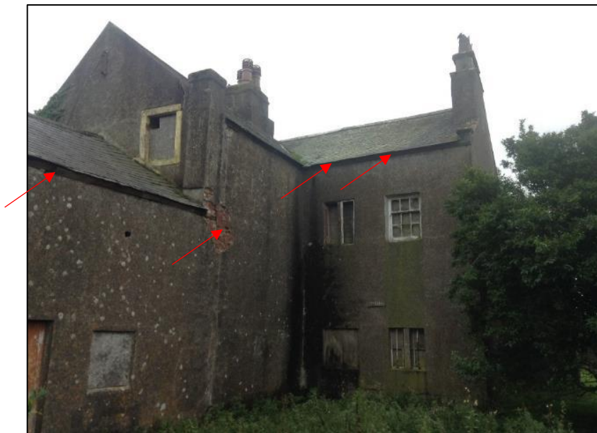
Photo 4: Western elevation of Building 1. Gaps in exposed brick work and at exposed stonework at soffits. A gap in the boarded-up window is large enough to allow barn owl and other birds to access the internal areas of the building.
