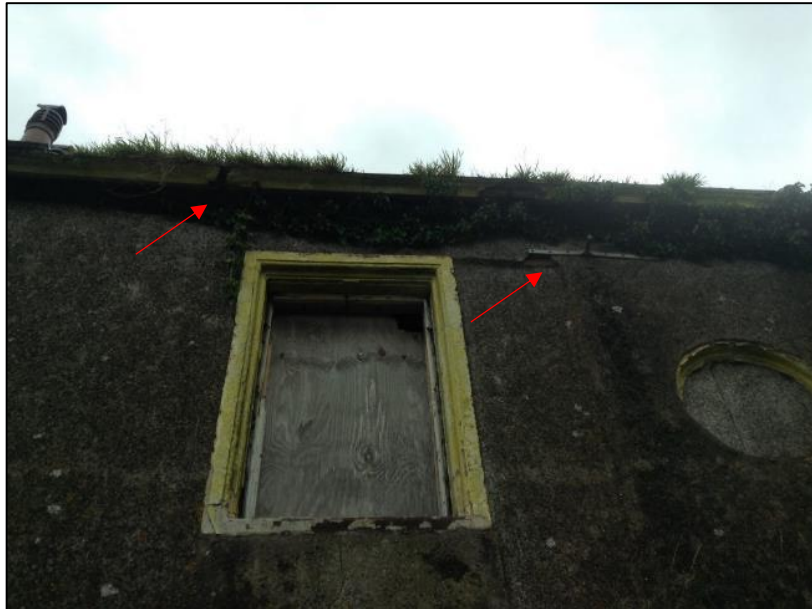
Photo 5: Eastern elevation of Building 1. Gaps in the soffit.
