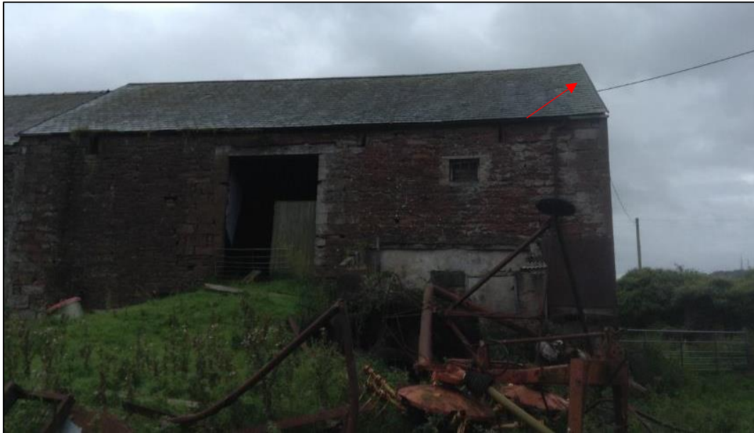
Photo 12: Northern elevation of Building 3. Numerous gaps in stonework and roof slates towards western gable (red arrow) provide potential roost features.
