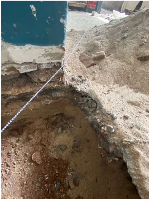
Left: Exposed floor to proposed kitchen.
