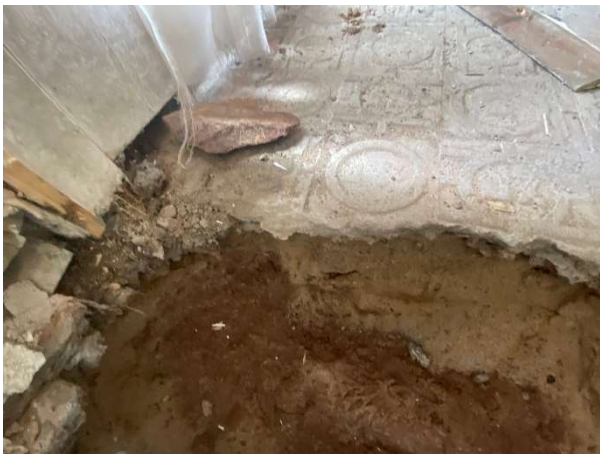
Left: Exposed floor to proposed utility
