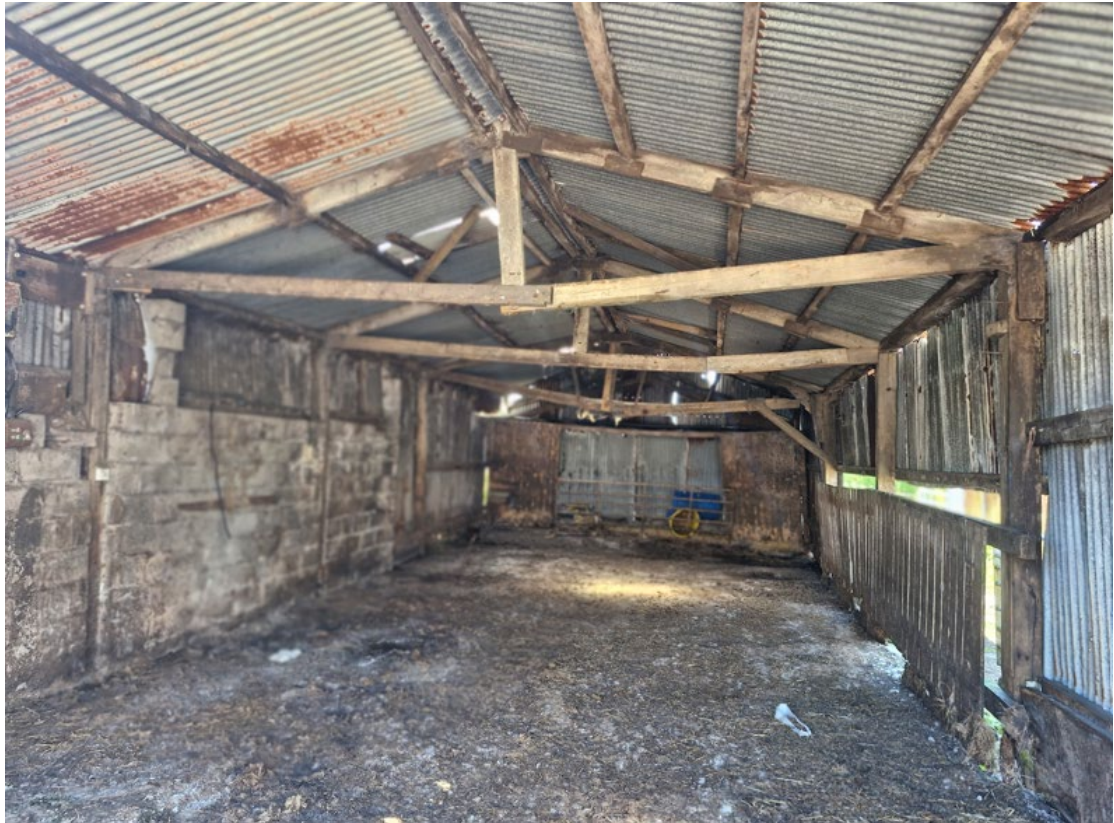
PHOTO 07 TIMBER PORTAL SHED TYPICAL INTERNALLY
