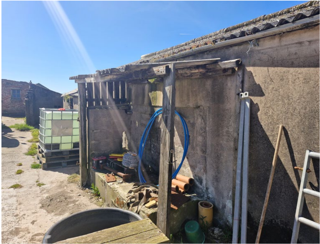
PHOTO 03 LEAN-TO CANOPY FRONT BUILDING
