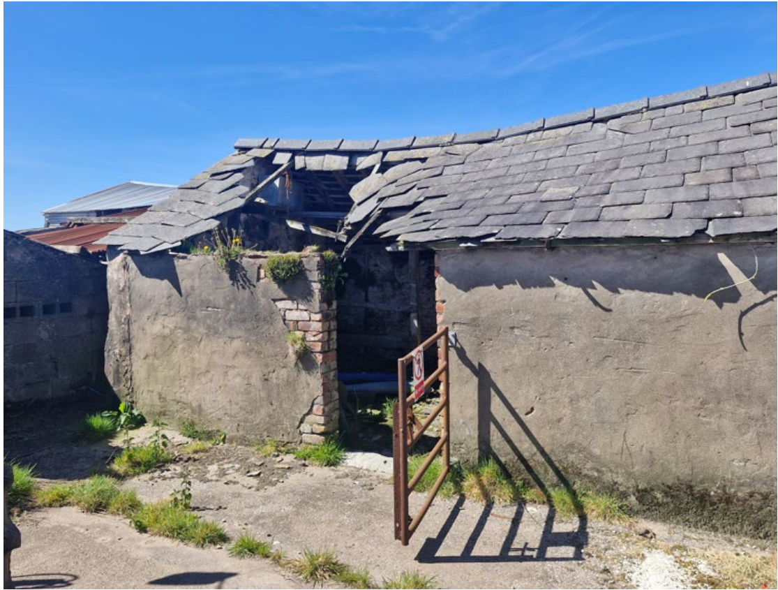
PHOTO 11 COLLAPSED ROOF
