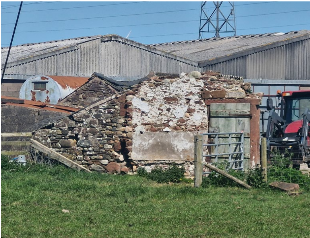
PHOTO 04 VIEW LEFT HAND MASONRY BUILDINGS
