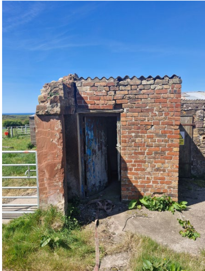
PHOTO 05 FRONT LEFT BRICK MASONRY BUILDING
