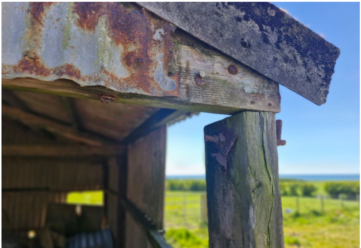
PHOTO 08 TIMBER PORTAL COLUMN/TRUSS CONNECTION (TYPICAL)
