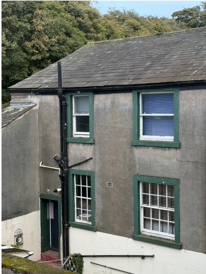
Side view from alley/next doors property
