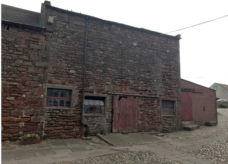
Figure 3.2 – Yard side wall of Barn One
