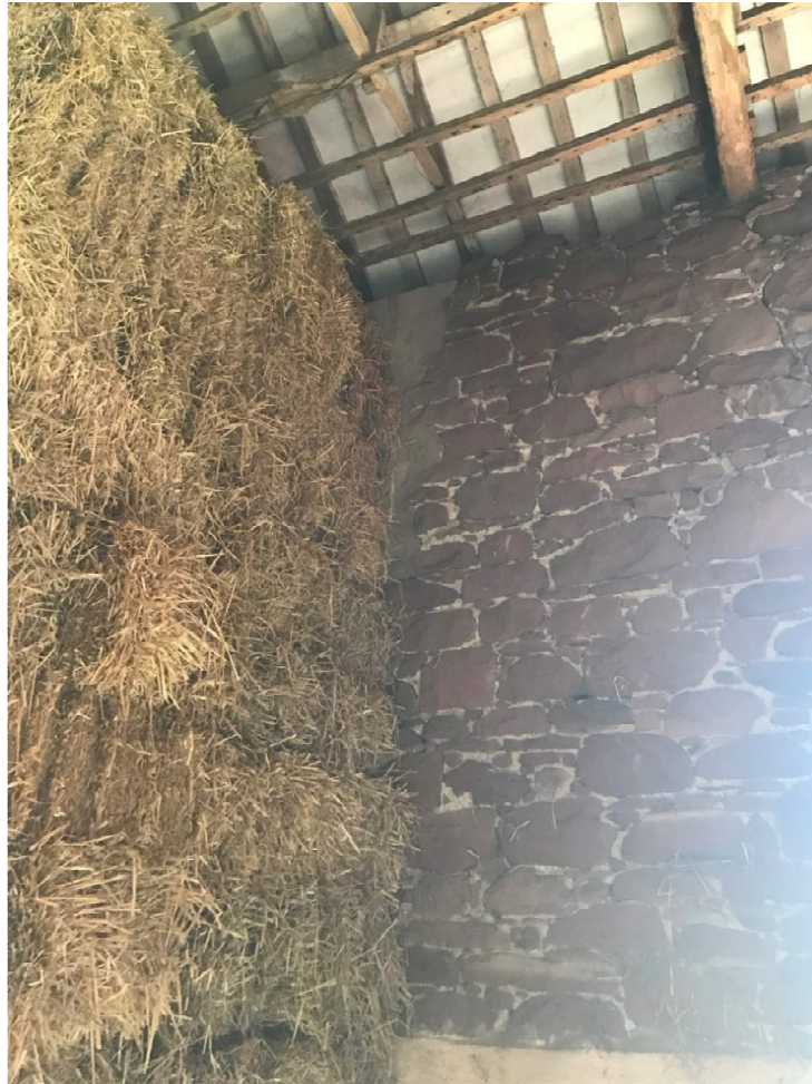
Figure 3.14 – Edge of blockwork rebuild
