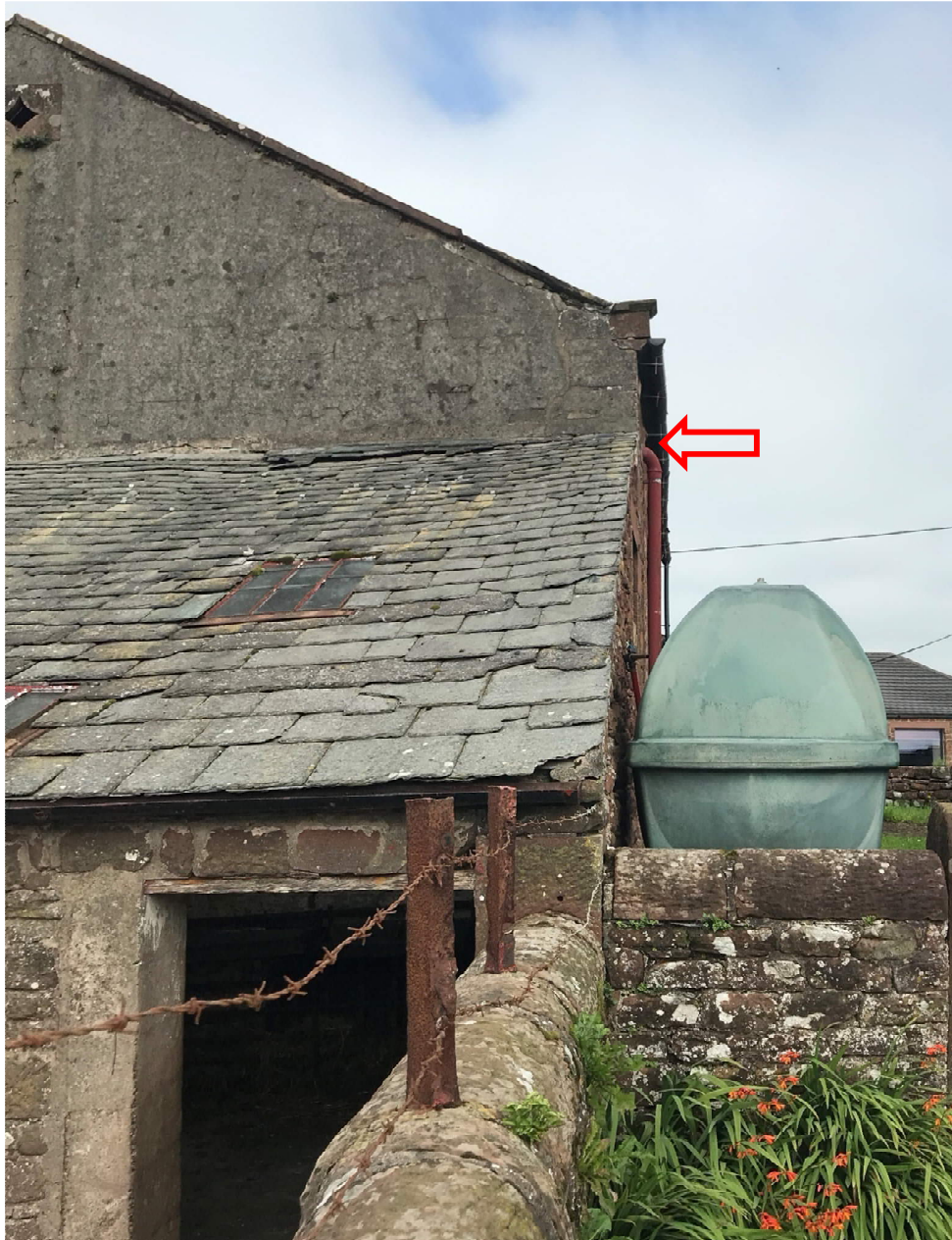
Figure 3.9 – Inwards dish in front wall
