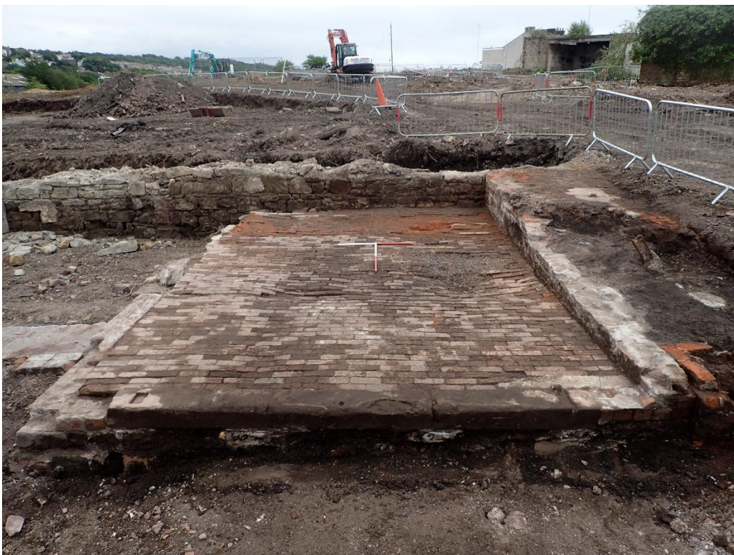
Photo 28: Area B, brick surface F93, looking south
