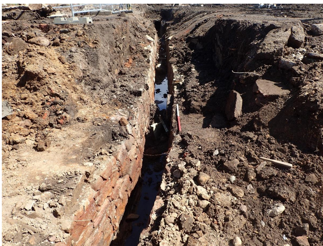
Photo 20: Area B, culvert F154 with the cap removed, looking south
