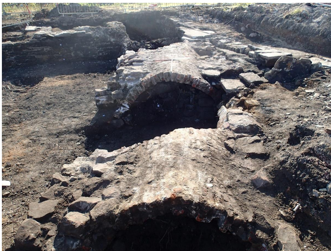
Photo 3: Area A, the tunnel, F67, F66 and F65, looking east
