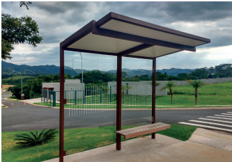
Bus shelter with green roof
