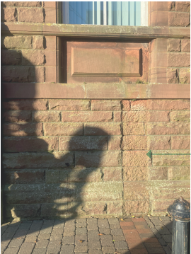
FIG 08 Site image showing the Town Hall building, viewed from the gap between this and the library. Here you can see a palmprint of the former wall that was used to stop pedestrians using the gap between the historic buildings as a through-route in the Town Square. The proposed link building will remove this route and direct all visitors and pedestrians through the new community hub, or through the refurbished public square.
