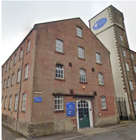
Image 3: Front Entrance off Earl Street.
