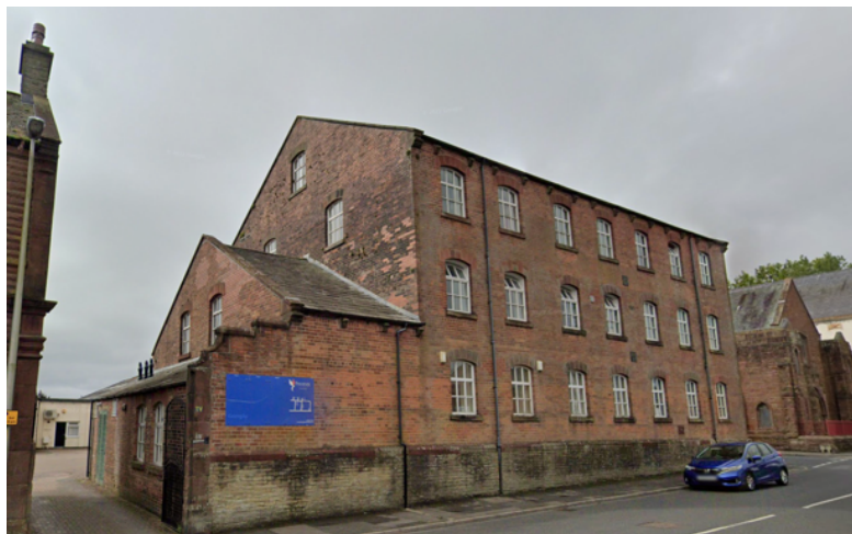
Image 4: Cragg Road Elevation with access into Phoenix Court, with two storey unit and single storey plantroom to rear elevation.
