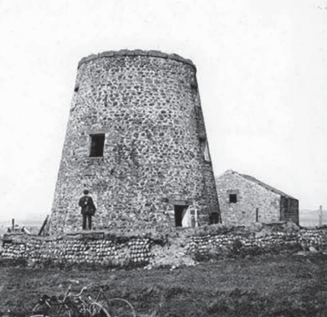
The Old Windmill, Walney Island with only masonry structure remaining (date unknown).
