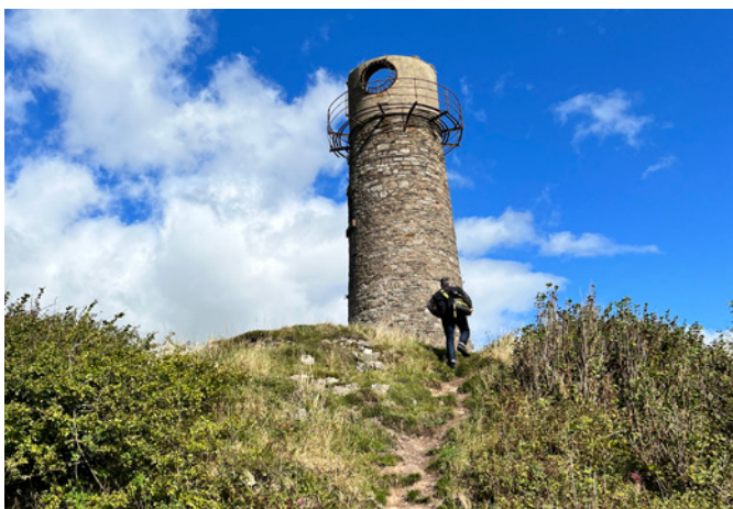
Poor access to heritage assets
