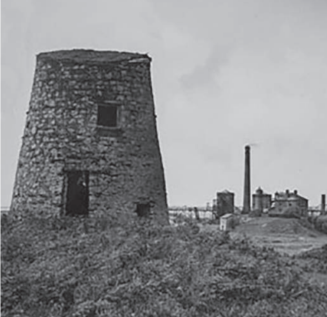
Towsey Hole Windmill with only masonry structure remaining (circa 1889).
