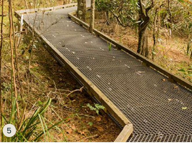
Raised Steel Walkway
