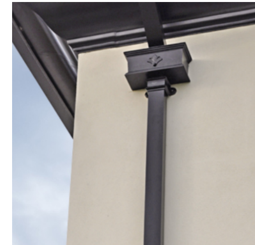
Heritage cast style aluminium rainwater pipes. Guttercrest or equal and approved.
