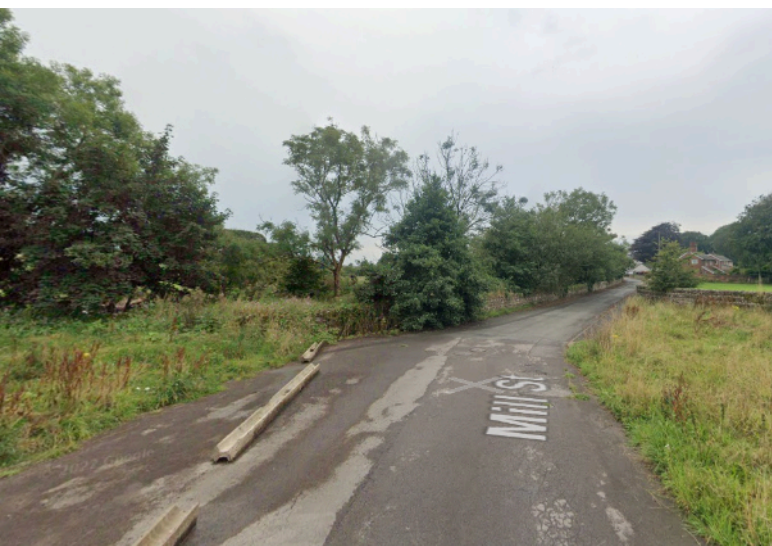
04 Rear access road facing Mill Street
