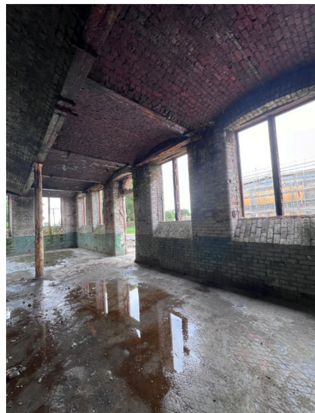
08 Internal view. Room with vaulted brick ceilings
