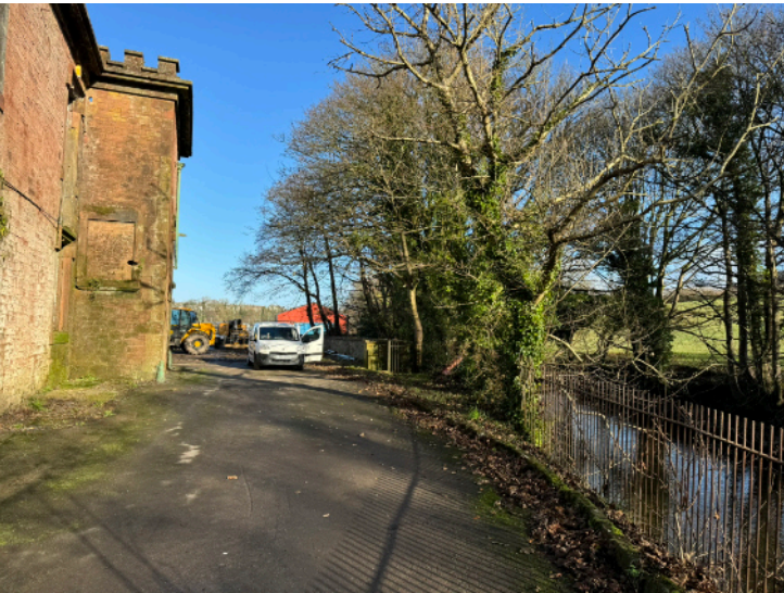
02 East elevation. View facing towards the river Ehen
