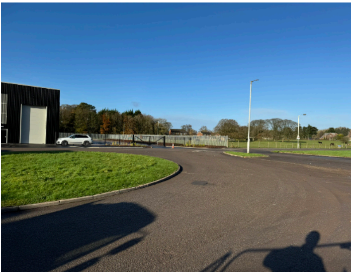
03 View facing towards the site entrance next to the roundabout and the new industrial and commercial unit to the west of the building.
