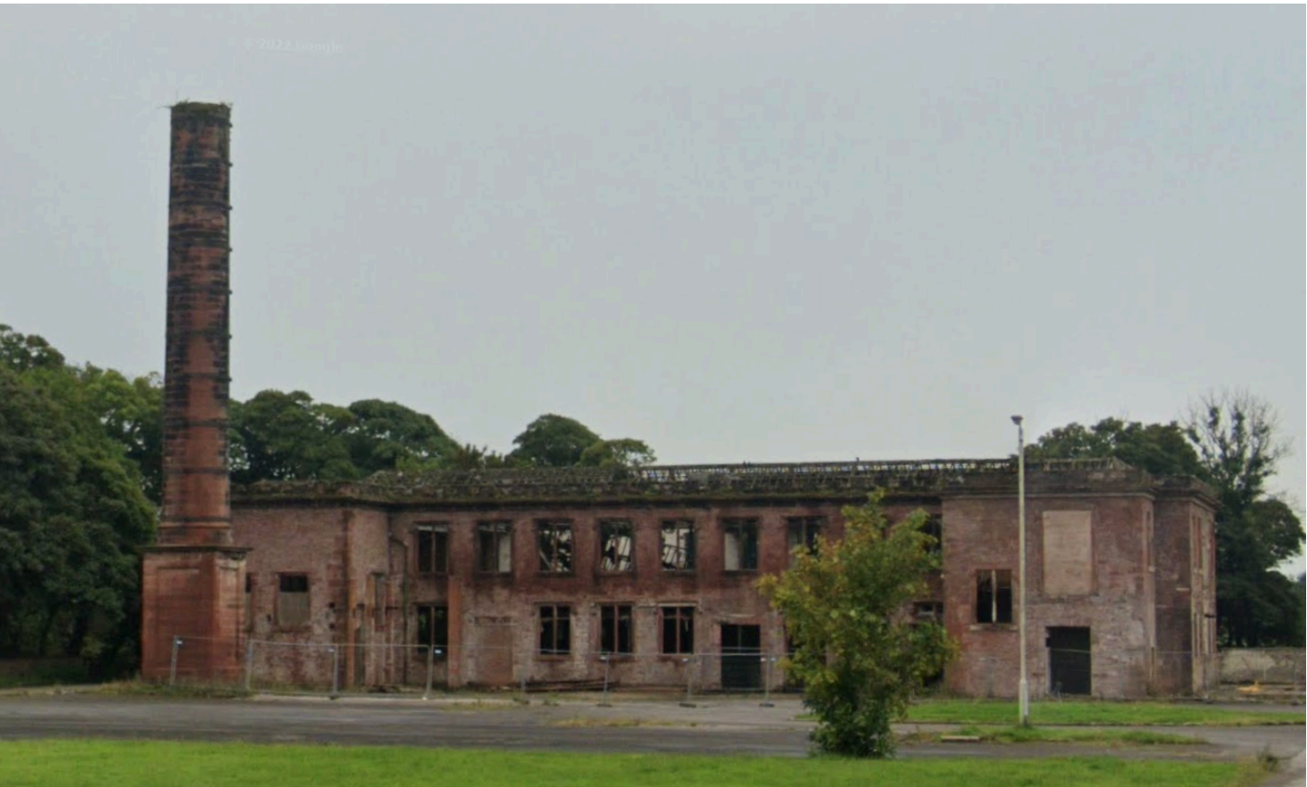
01 North building elevation also showing the redundant chimney
