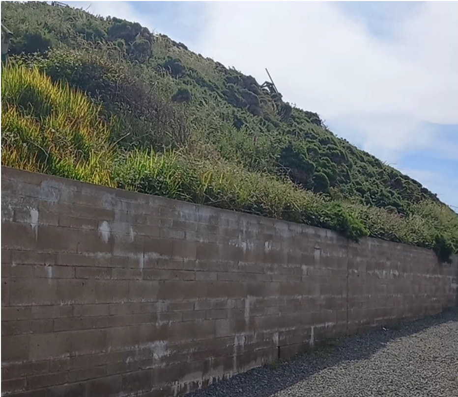
View South-East from the Public Footpath
