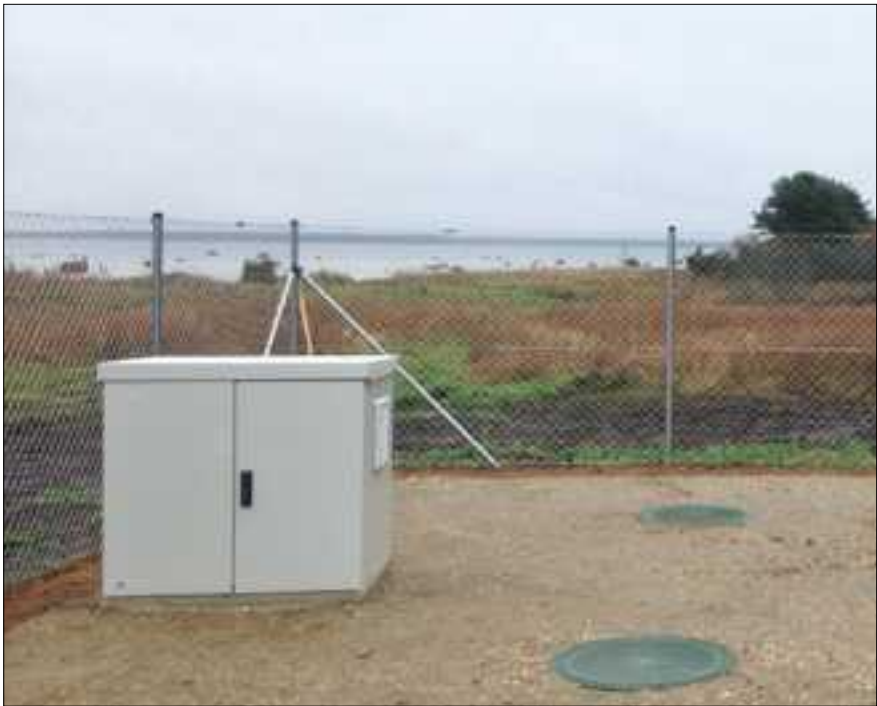
The image shows the External steel cabinet XL for 50 inhabitants
