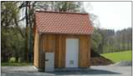
Example: Installation in a machine house
