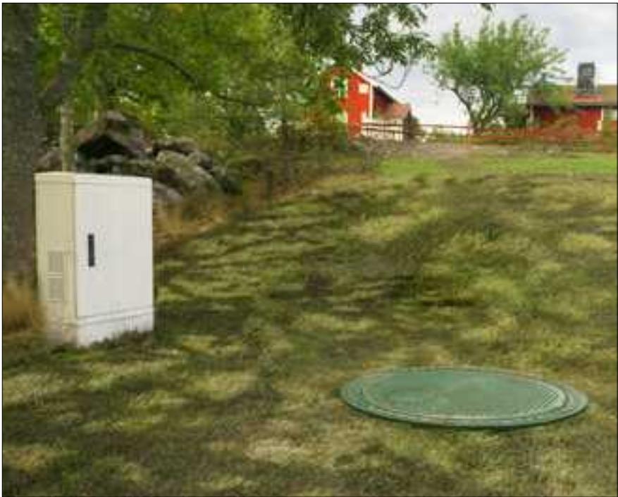
The image shows the External plastic cabinet L with LED warning light for 20 inhabitants
