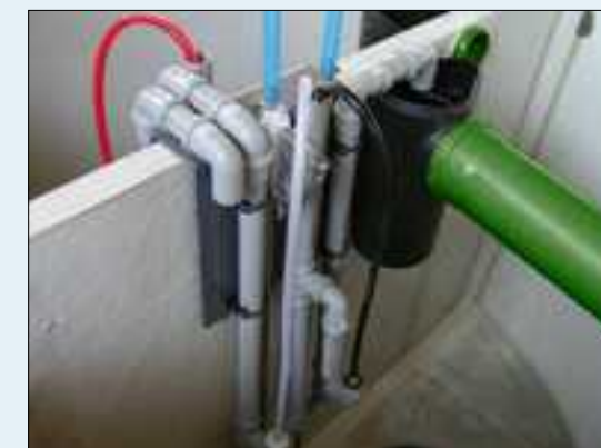
Image shows System pack for retrofitting > 28 inhabitants)
