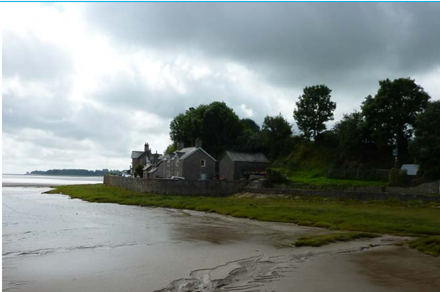
Figure 5-2: Masonry wall at Hammerside Hill (top). Short recurve wall to the north of Hammerside Hill (middle). Earth embankments south of Flookburgh (bottom).
