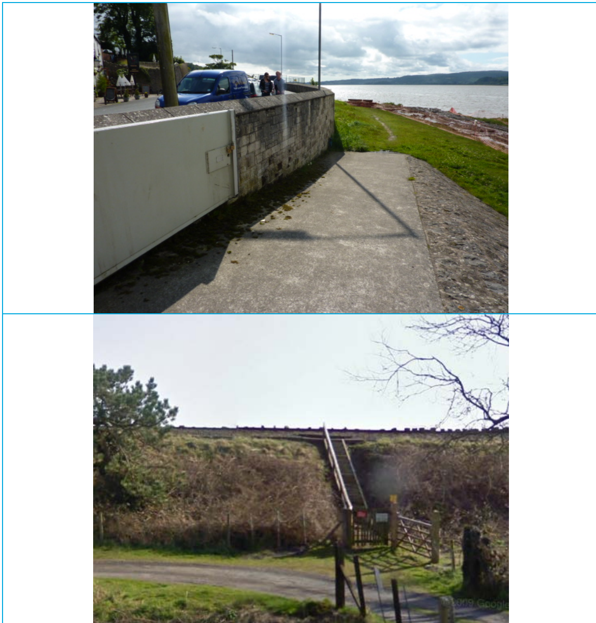
Figure 4-2: Flood wall and pedestrian access flood gate at Arnside (top). Railway embankment along Meathop Road (bottom)
