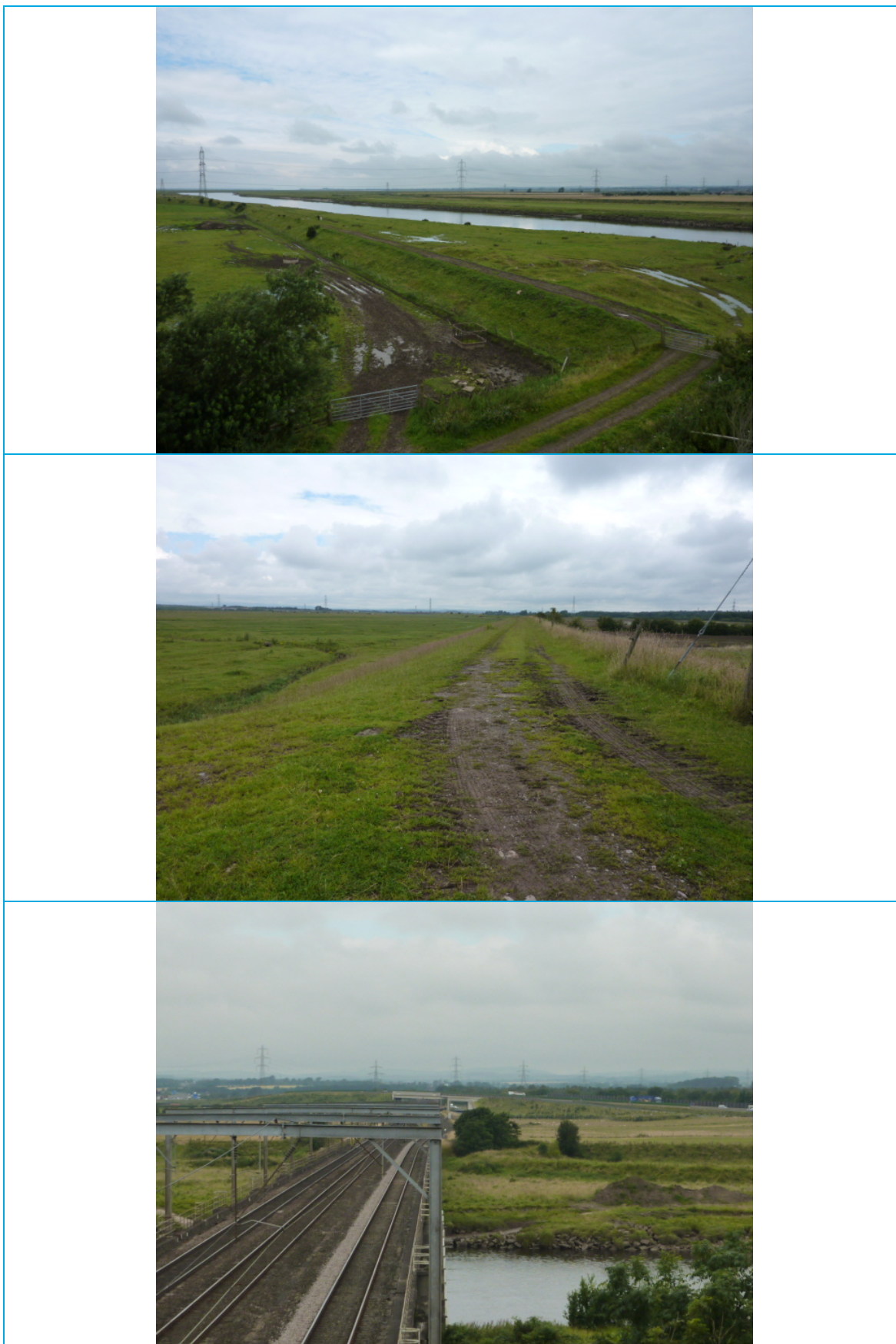
Figure 13-2: Earth embankments at Metalbridge on the Esk (top). Embankment running across Rockcliffe Marsh (middle). Railway line and M6 motorway infrastructure (bottom).
