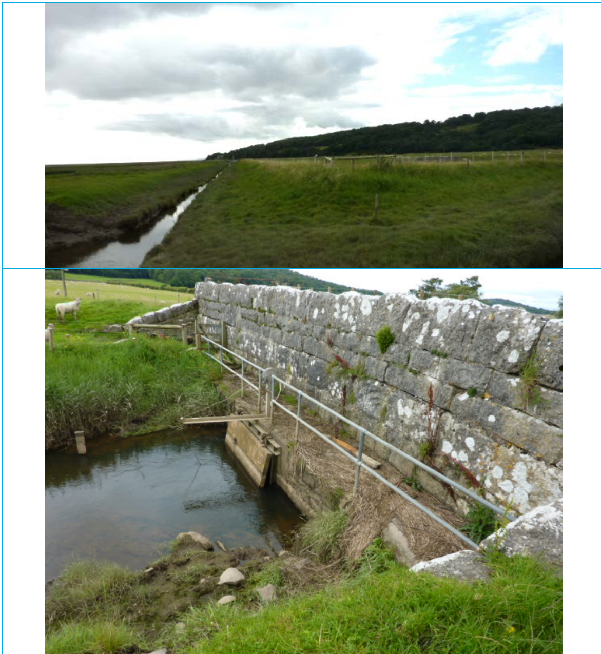
Figure 3-2: Earth embankment at Quicksands Pools (top). Tidal flap at Quicksands Pool Drain (bottom)
