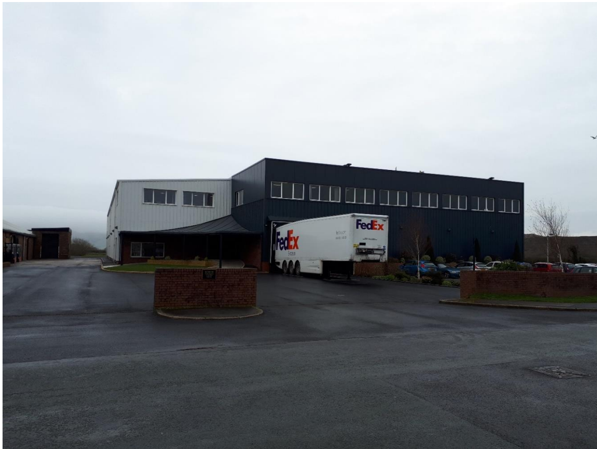
Photo 1/2 – Existing Main Entrance (West Elevation)
