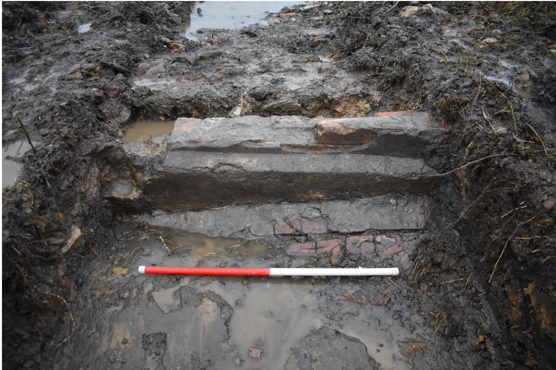
Fig.6 - Photograph of E-W Orientated Wall (602)
