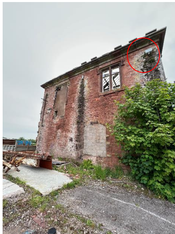
Image 2. Western aspect of B1, with bat entry point highlighted.
