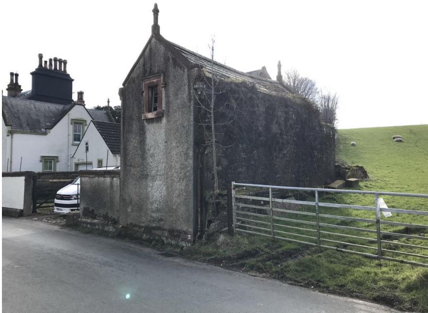
View away from Barwickstead showing barn built into hillside. Vegetation growths to stonework require removal
