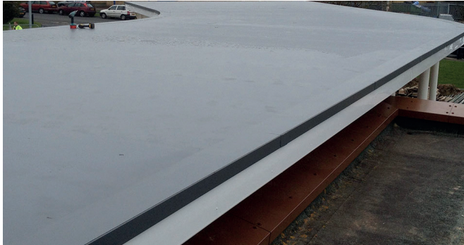
Single ply roofing
